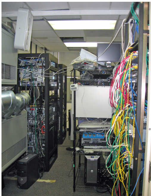
Figure 4.27: View of server and graphic work stations in Room 218 used by the Bioinformatics Center. Note the cooling service on the left required to keep the systems functioning. Courtesy of Michael Feig.
