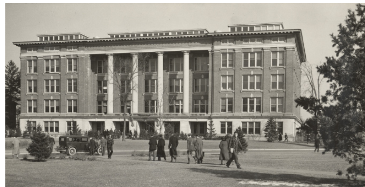
Figure 1.6: Agriculture Hall built in 1909 (Stanford and Dewhurst 2002). Courtesy of the Michigan State University Archives and Historical Collections (MSU Buildings, Agriculture Hall folder).
