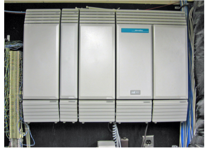
Figure 4.24: Meridian Norstar Computer in the basement of the Biochemistry Building for the Department's Digital Phone System. Courtesy of Ron Norris.
