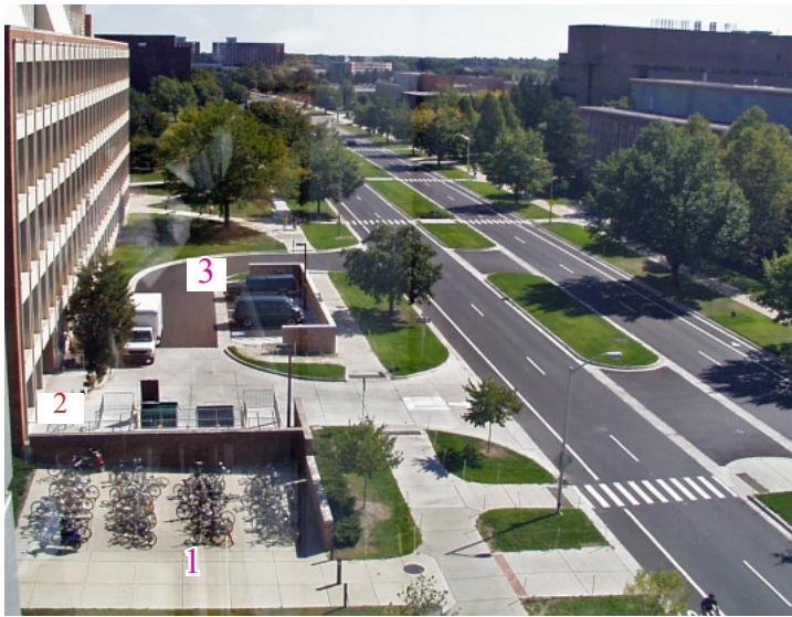
Figure 3.7: View of the redesigned parking area on the south side of the Biochemistry Building in 2007. The view, looking east along Wilson Road, first shows (1) a bicycle parking area, (2) the loading dock and (3) the entrance to the area. UA 16.18, Michigan State University Archives and Historical Collections, East Lansing, MI.
